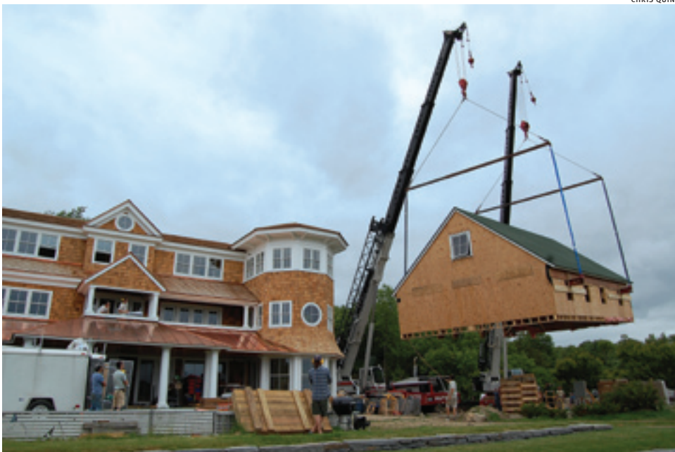
To open up an expansive view of Lake Champlain and the Adirondacks, the three-bay garage was lifted off its slab and moved from one side of the house to the other.
