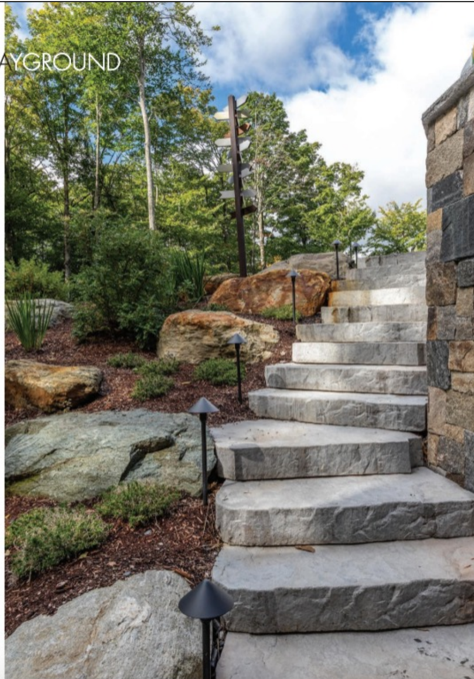
THE STEPS UP from the bathroom shower area to the pool are actually concrete made to resemble real stone. The color was selected to integrate well with the stone veneer on the retaining walls and the boulders in the garden.
